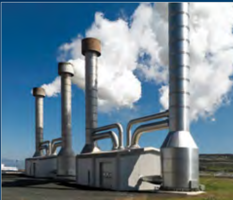
Geothermal Energy Studies
