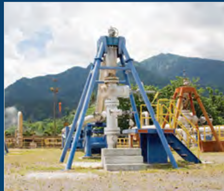
Geothermal Well Testing
